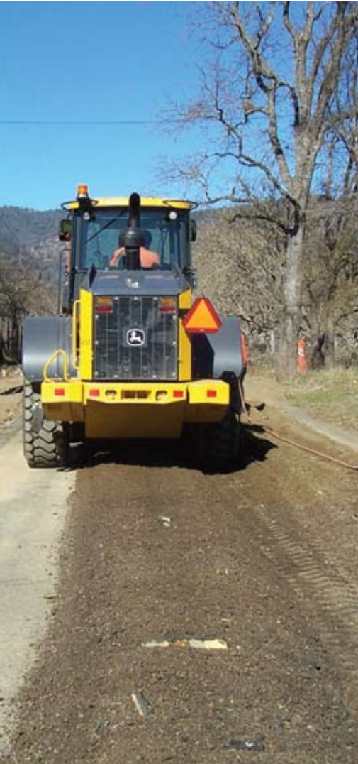
Lake County Crews prepping replacement bridge approach
