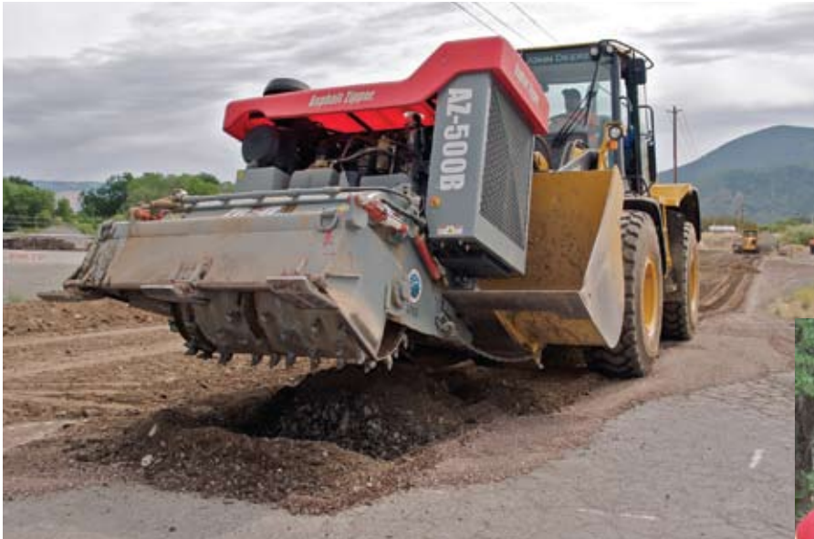
Lake County (California) uses its Asphalt Zipper unit both for road patching and, occasionally, to recycle an entire roadway (left). Below, Lake County Crews performing FDR for road reconstruction.
