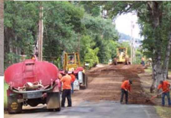
Lake County (California) uses its Asphalt Zipper unit both for road patching and, occasionally, to recycle an entire roadway (left). Below, Lake County Crews performing FDR for road reconstruction.
